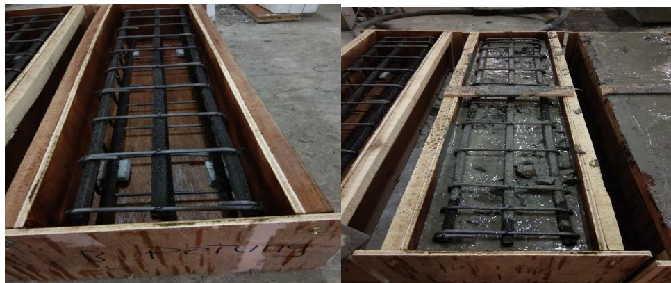
Figure 4: Making formwork
