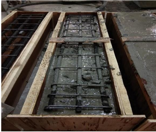
Figure 5a Casting process
