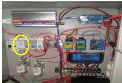
**Gambar 10.** Schneider Miniature Circuit Breaker
