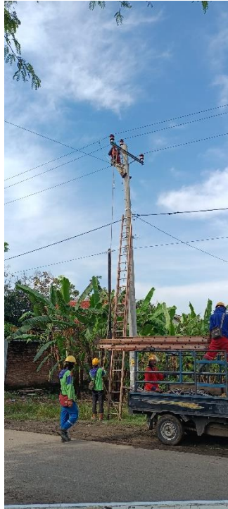
Gambar 4. Proses Pemasangan Jumper
